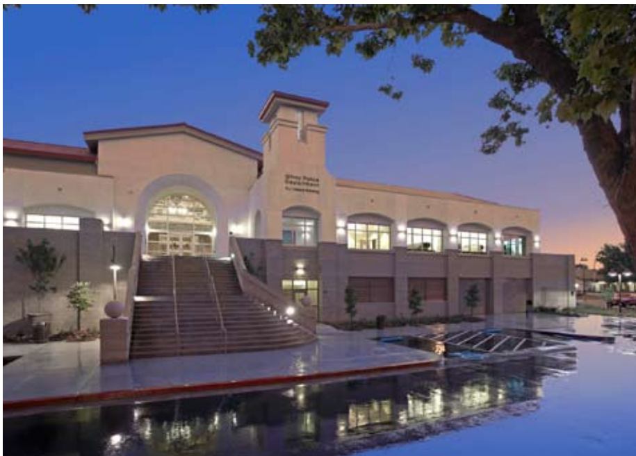
The new police facility was completed in January 2007 and used a total of 15,000 square feet of Met-Tile panels in a Mission Clay color.
